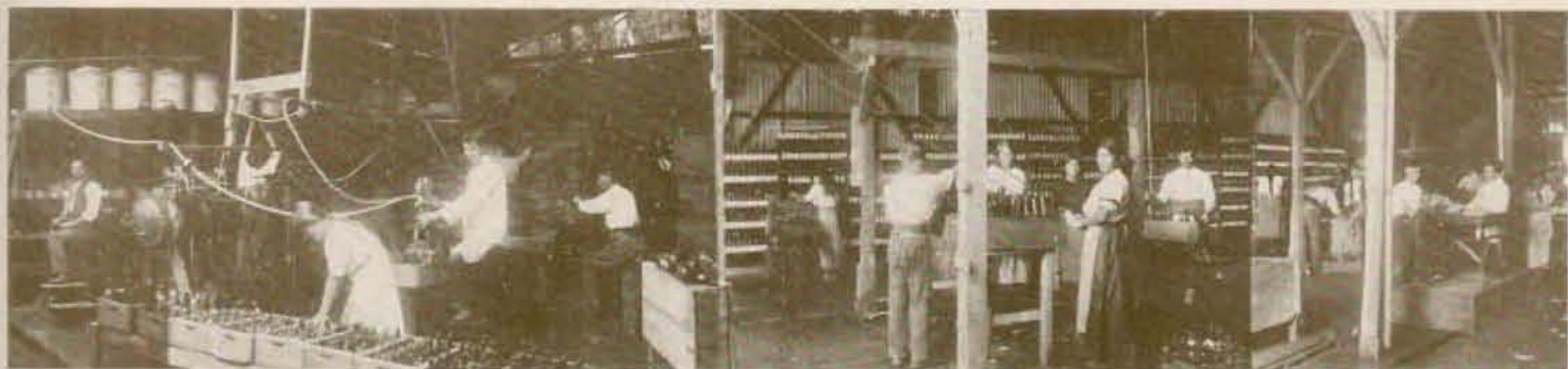
VISTA GENERAL - INTERIOR - GENERAL VIEW
